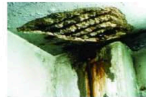
Fig. 1. Corrosion of reinforcing steel is the most common cause of concrete deterioration. (46080)
